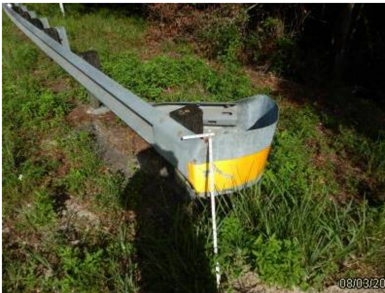
Photo 5 - Element 8099 PS Conc Slab (Sonovoid)
