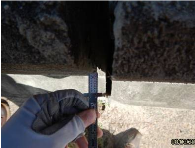
Photo 7 - Element 8099 PS Conc Slab (Sonovoid)
