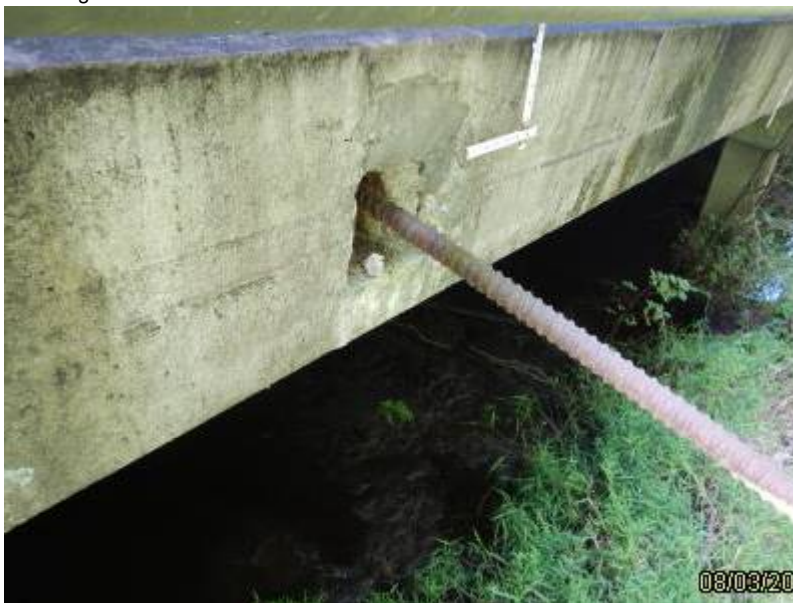
Photo 2 - Element 8099 PS Conc Slab (Sonovoid)
