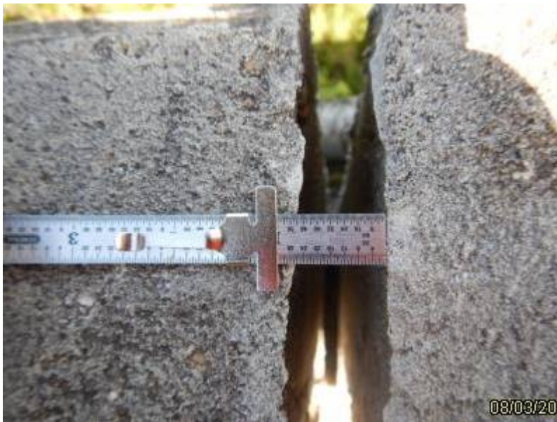
Photo 8 - Element 8099 PS Conc Slab (Sonovoid)
