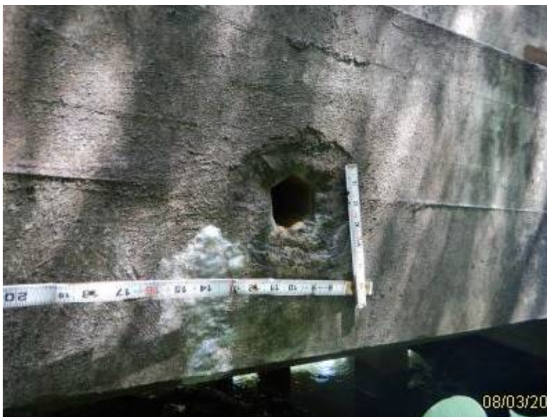
Photo 1 - Element 8099 PS Conc Slab (Sonovoid)
