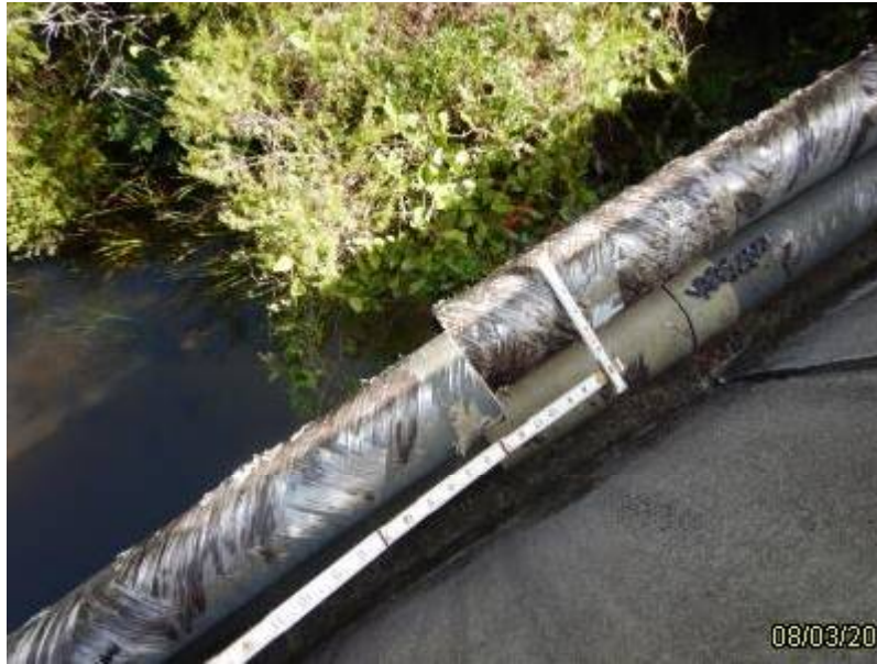
Photo 9 - Element 8099 PS Conc Slab (Sonovoid)
