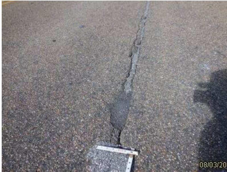
Photo 11 - Element 8099 PS Conc Slab (Sonovoid) (510 Wearing Surfaces)
