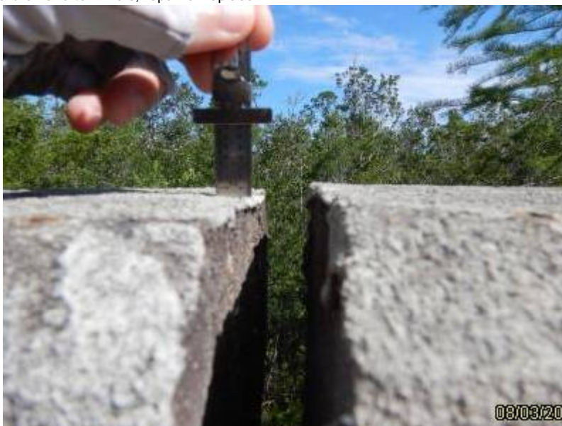
Photo 6 - Element 8099 PS Conc Slab (Sonovoid)
