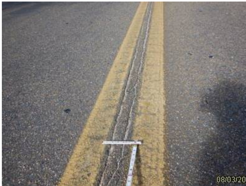
Photo 10 - Element 8099 PS Conc Slab (Sonovoid) (510 Wearing Surfaces)
