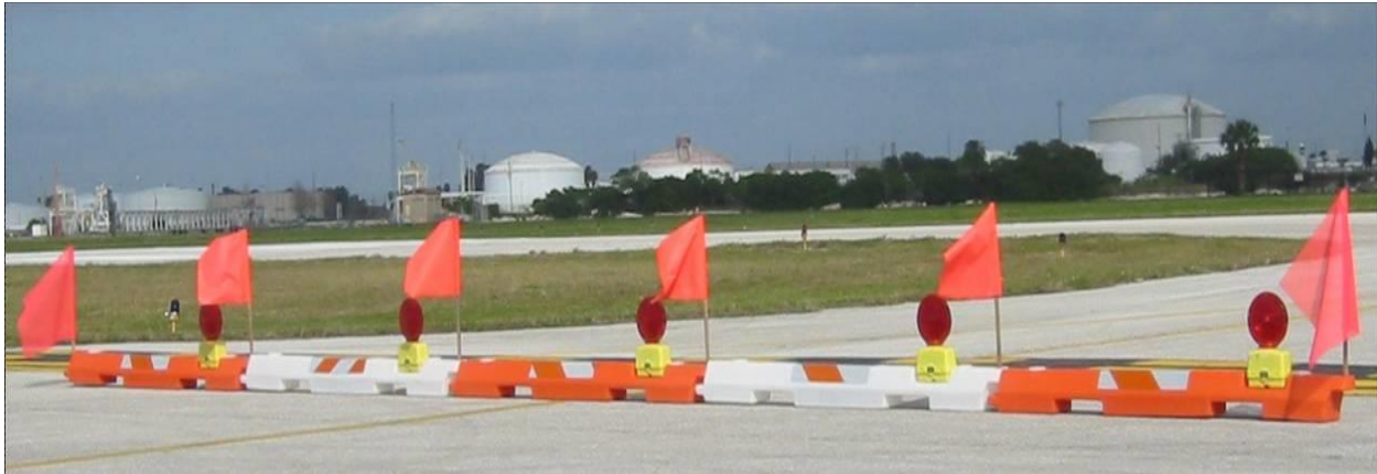
Figure 2-8. Interlocking Barricades
