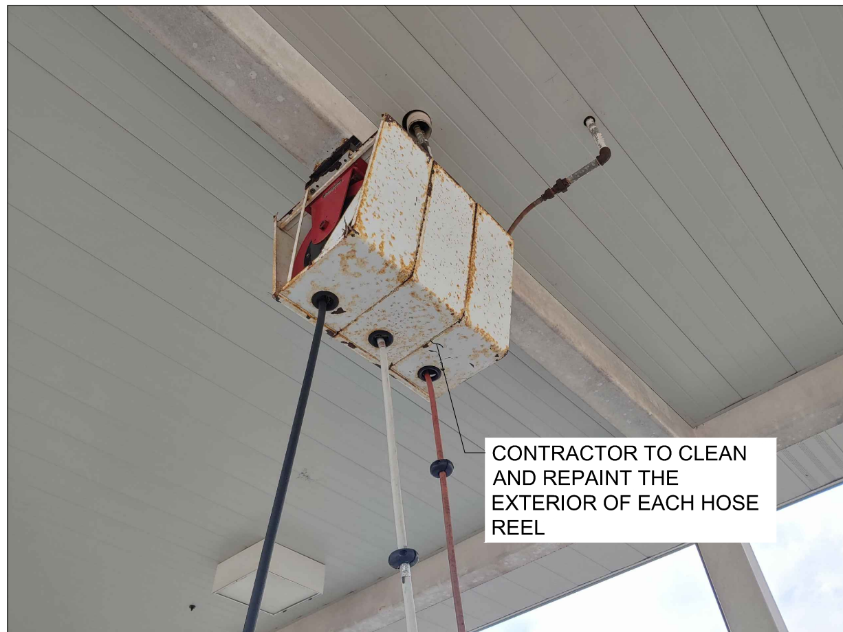
CONTRACTOR TO CLEAN AND REPAINT ALL EXIST. STEEL STRUCTURAL COMPONENT OF THE FUEL ISLAND FACILITY (MATCH EXIST. COLOR)
